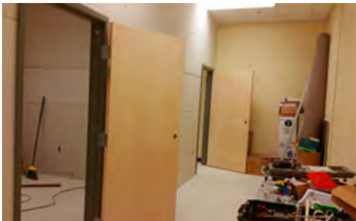
Construction of the SBHC space at North Central High School.
